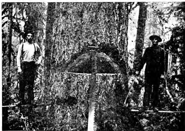
FIG. 21. — The Undercut on a Douglas Fir Tree. The fallers are standing on spring boards to enable them to make the cut above the root swelling. Washington.
